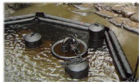
f) Pump skimmer (Source: Ro cleandesmi)
